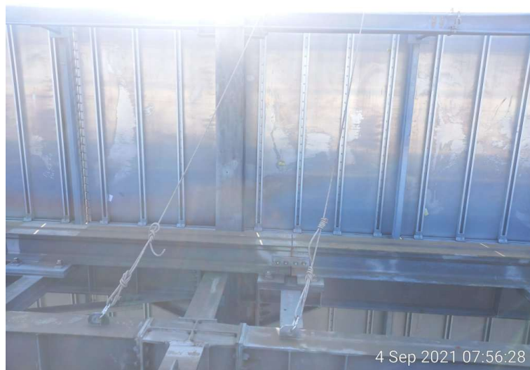
Photo 27. Tali Pengaman Minimum Kapasitas Beban Tarikan 500kg. Life Line Minimum Safe Work Load Capacity 500kg.
