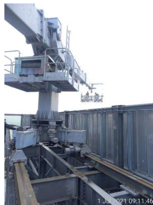
Photo 16. Gondola & Permanent Relnya. The Gondola & Its Permanent Rail
